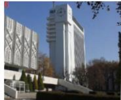
6 NAME: TYPOGRAPHIES BUILDING YEAR: 1974 ARCHITECTS: BLEZE R., GORBENKO A., VLADIMIROV L., GIBNO O., KRISTICH L.
