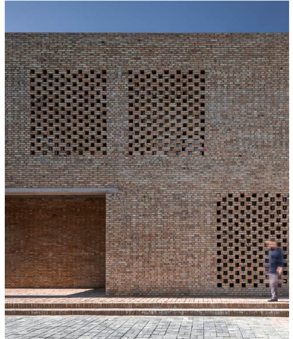
Sanhe Village Community Center, Sanhe, 2018
