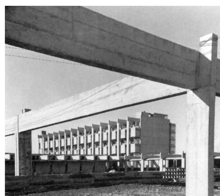
Exterior space defined by structure
